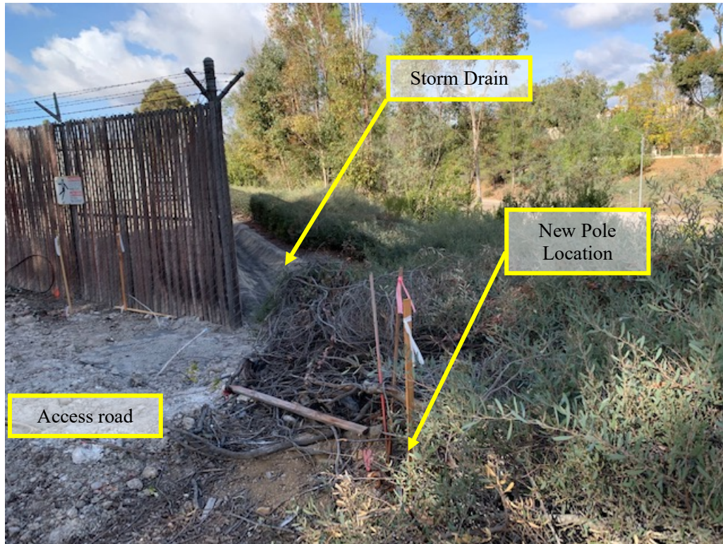
Photo 3. View of storm drain location west of Location 64 (E24). Best Management Practices (BMPs) are recommended to avoid construction debris and sediment entering the storm drain. View northwest.
